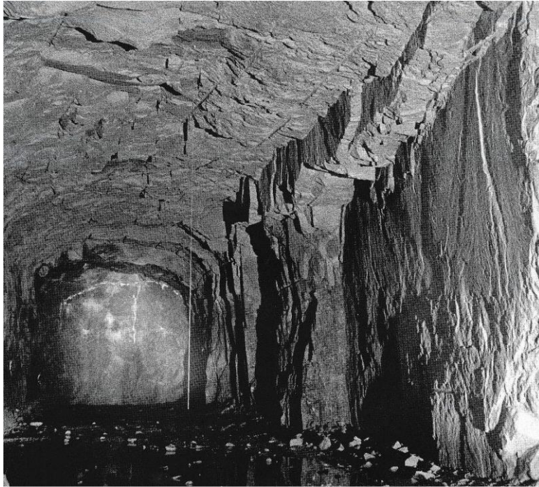
Figure 5: Slabbing and slickensiding caused by large shear strain can give the rock mass strongly anisotropic hydraulic and mechanical properties (After Morfeldt).
