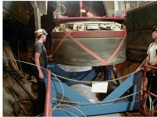
Figure 8: Two repository concepts showing the entities that determine stability and risk of pollution. Upper left: The KBS-3 concept for disposal of HLW in copper/iron canisters surrounded by dense blocks of smectite-rich clay. Lower left: Placement of 2,000 kg clay block. Upper right: disposed LLW or ILW cast in concrete and embedded in effectively compacted granular smectitic clay. Lower right: On-site compacted granular smectitic clay before final rounds by ordinary rollers (Pusch et al, 2017).
