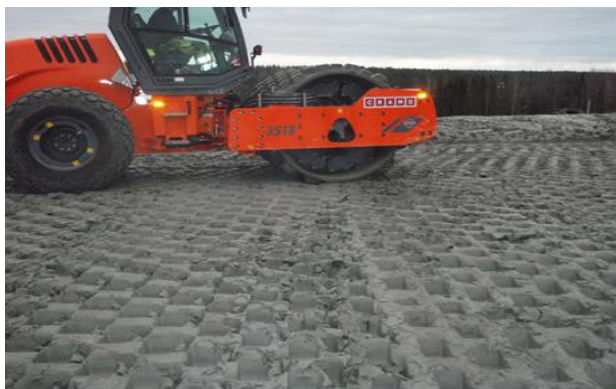
Figure 28: Vibrating padfoot-roller on compacted natural clay with about 20% water content.
