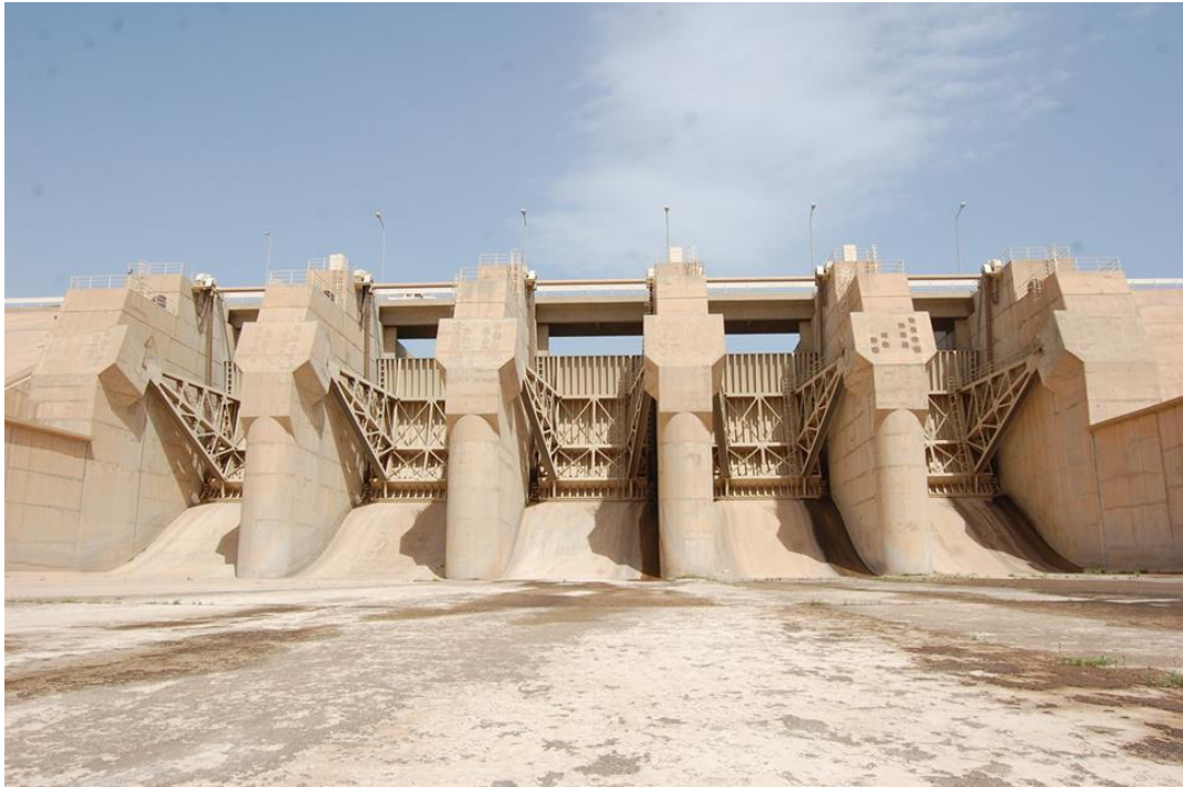
Figure 14: Spillway gates of Hemrin Dam, view from the downstream. (Source:[6]).
