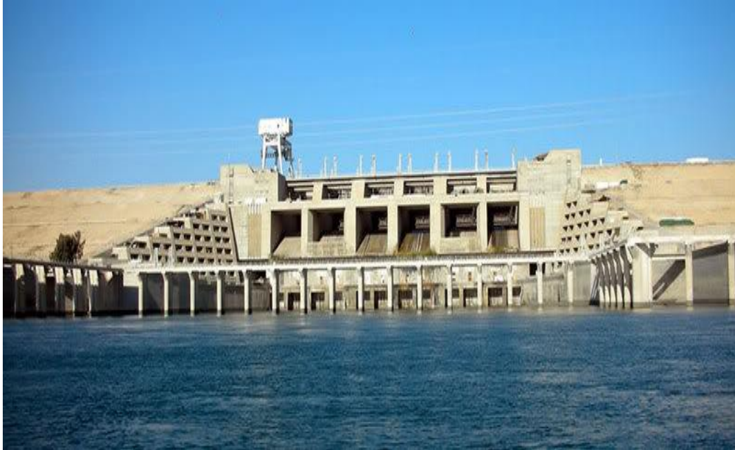
Figure 16: Concrete Section of Haditha Dam, view from the downstream. (Source:[6]).
