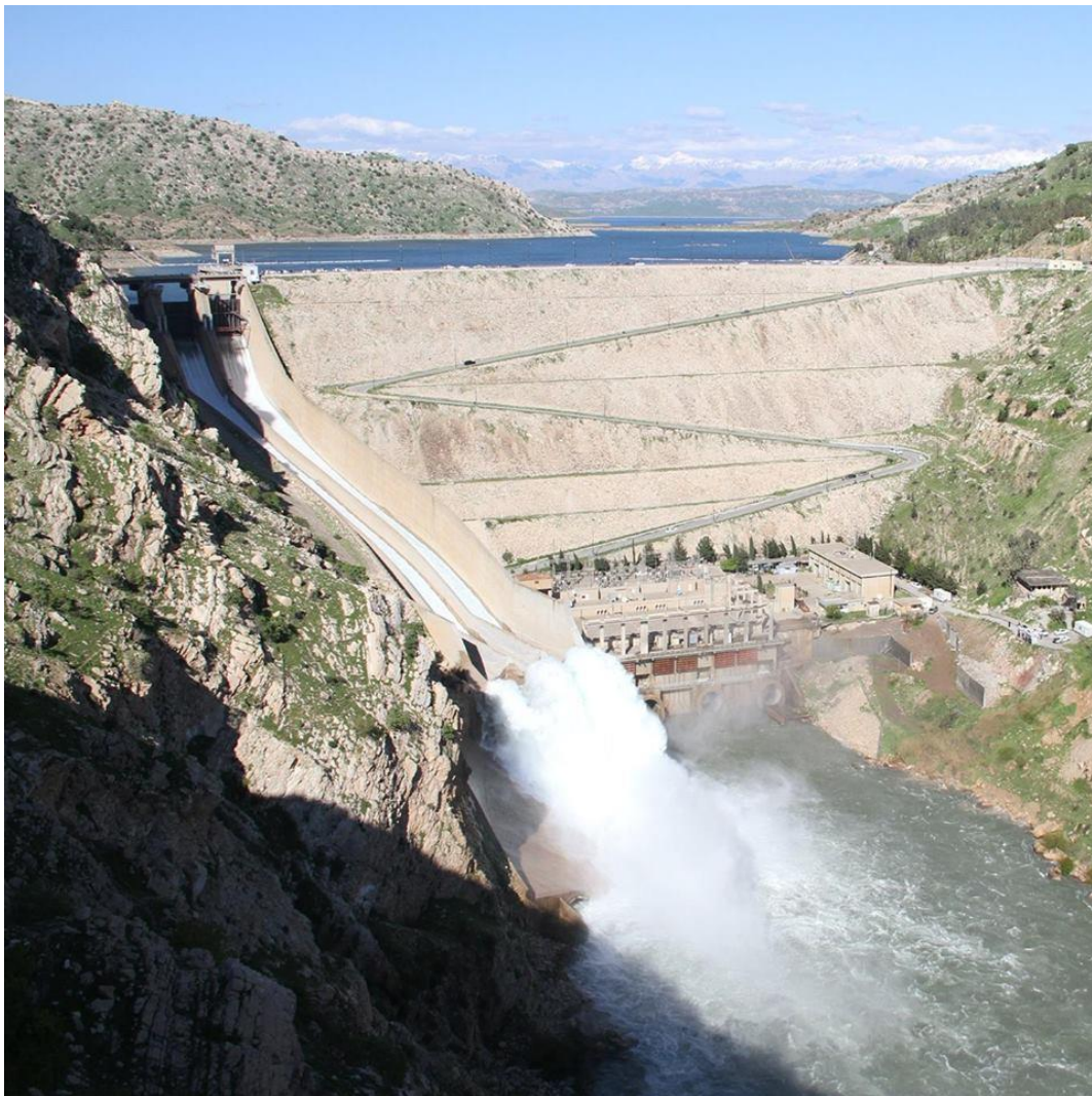
Figure 10: General view of Darbandikhan Dam from the upstream. (Source:[6]).
