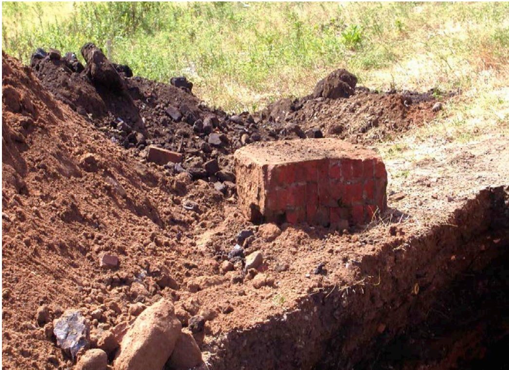
Figure 3: Shallow excavation showing fills comprising discarded construction materials.
