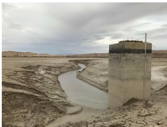
Figure 3: General view of Mandaly Dam Reservoir filled with sediments [12].
