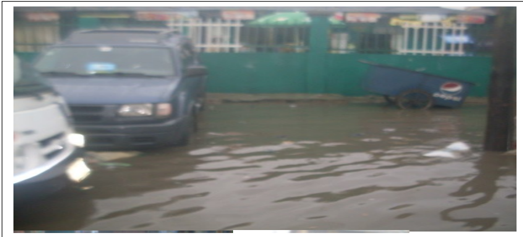
Figure 5: Flooded building in the Study Area
