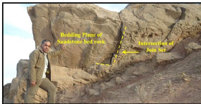
Figure 6: Intersection of joint sets and bedding planes of sandstone bed.
