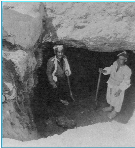
Figure 32: Photograph showing the Excavation of Bavian tunnel [10].
