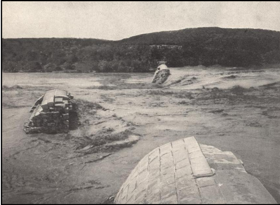
Figure 21: A view of the dam one hour after break [32].
