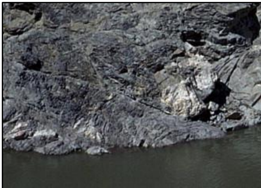
Figure 15: Close view of a cross section of the main fault on right bank. The finely crushed borders of the fault zone are well visible.
