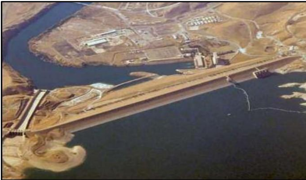
Figure 8: Aerial view of the Main Mosul Dam and appurtenant structures.
