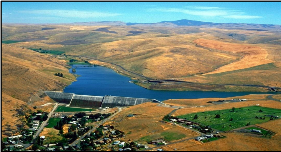
Figure 13: View of Willow Creek Dam [12].
