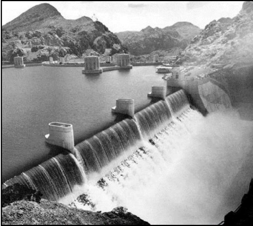
Figure 27: Water from Lake Mead discharging over the four drum gates of the Nevada spillway during spillway tests in August and October 1941.
