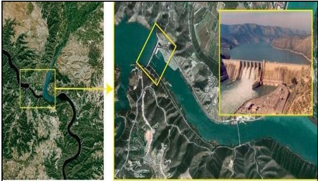
Figure 13: Left: Location of Mequinenza dam. Right: Downstream face of the dam.
