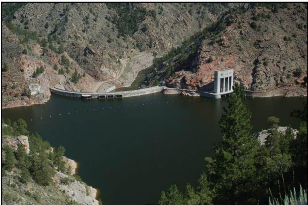
Figure 8: Upstream view of Seminoe Dam.
