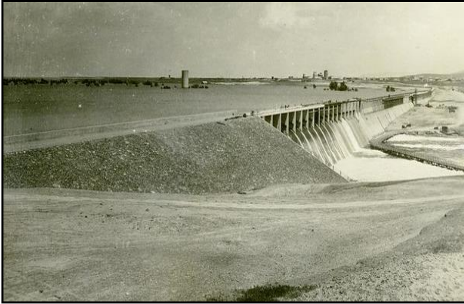
Figure 2: View of the old original American Fall Dam (1927).
