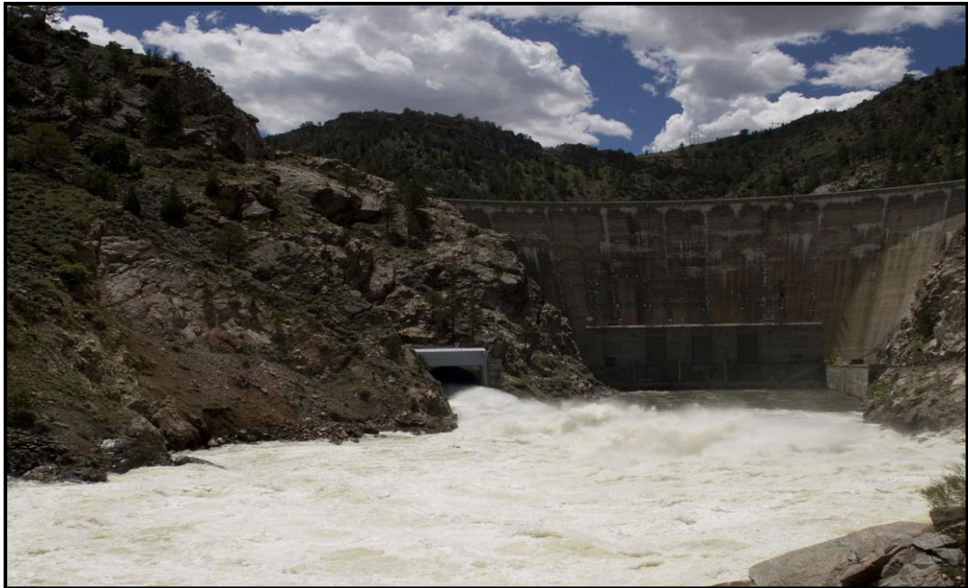
Figure 7: Downstream view of Seminoe Dam.
