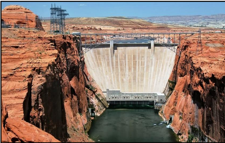
Figure 22: Downstream view of Glen Canyon Dam showing the Power Station and outlets of the two tunnel spillways.
