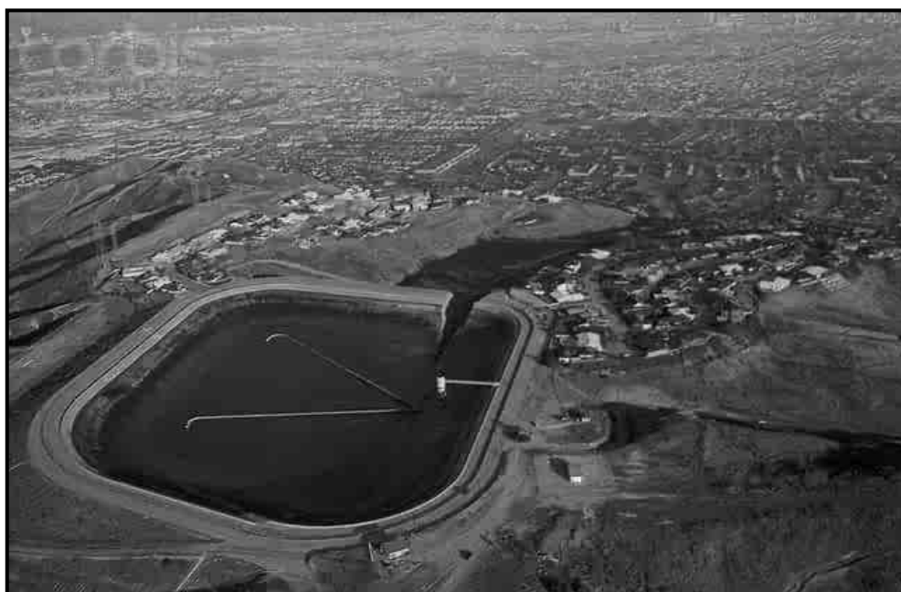
Figure 3: Aerial view of Baldwin Hill Dam Reservoir showing breaching section.
