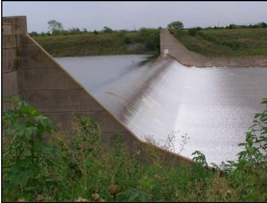
Figure 12: Lewisville Dam: view of spillway Ogee Weir looking east.
