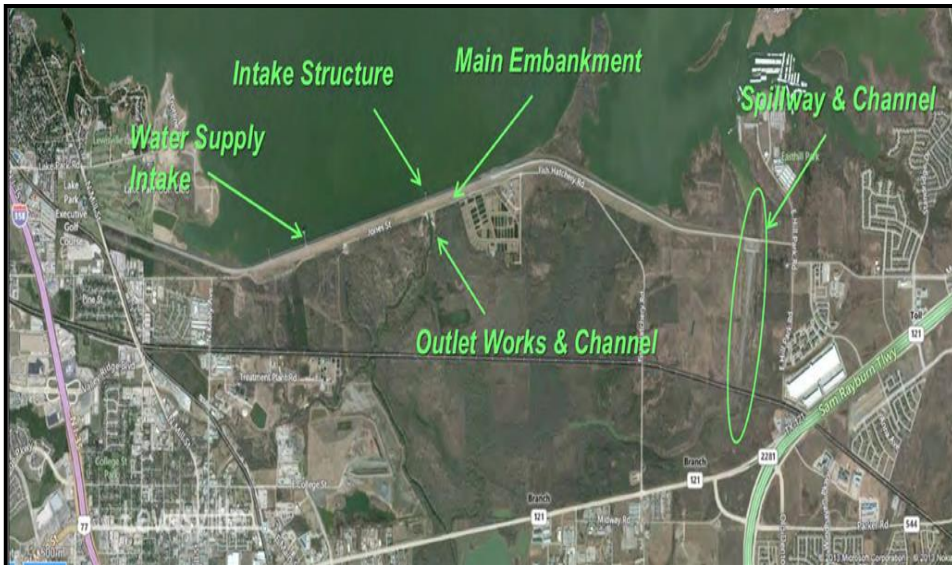
Figure 13: An aerial view of Lewisville Dam indicating the various components of the dam.
