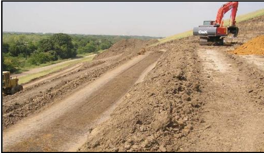
Figure 23: Fine materials used in the construction of the embankment.
