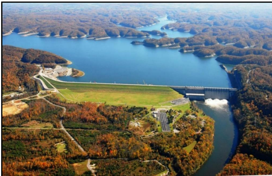
Figure 5: Overview of Wolfe Creek Dam, showing both concrete part and embankment.
