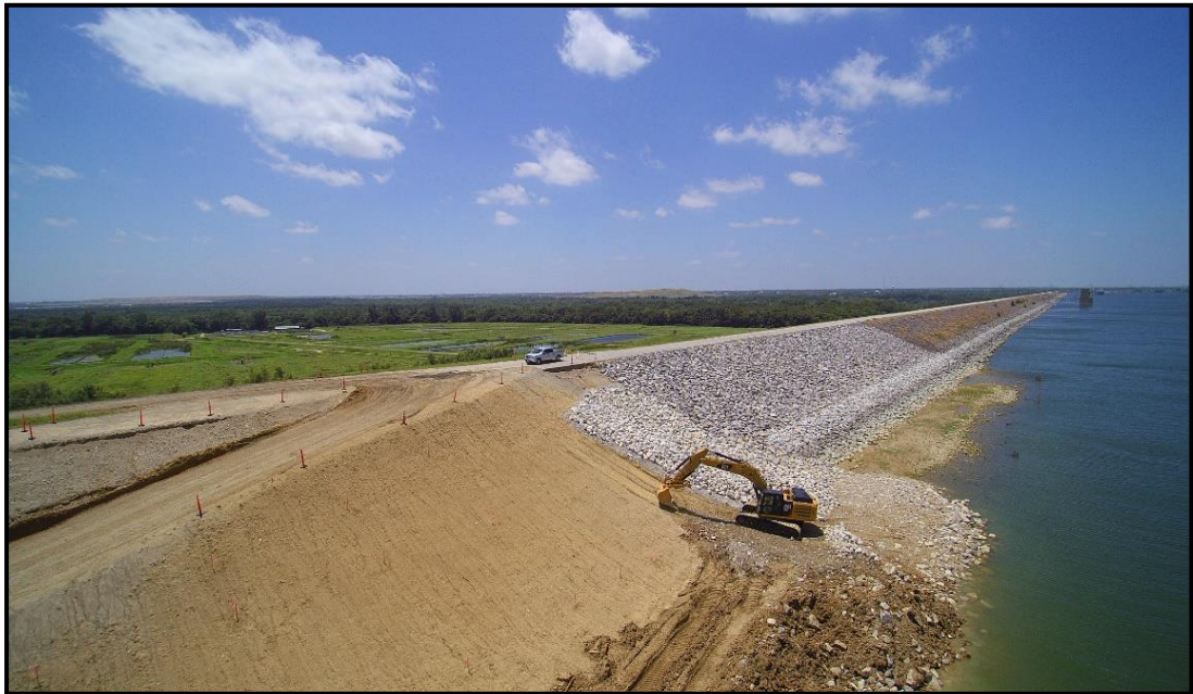
Figure 20: Repair work progressing on the slope of Lewisville Dam slide during 2016 [22].
