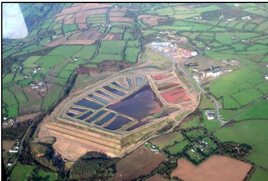
Figure 1: Aerial view of Wheal Jane tin mine Tailings Dam [9].
