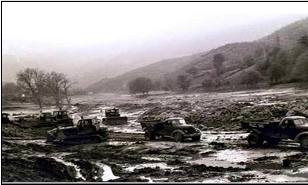
Figure 22: Cleaning operations in the flooded downstream Area [45].
