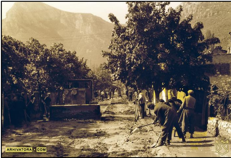
Figure 21: Cleaning of Zgorigrad streets from the toxic mud [45].
