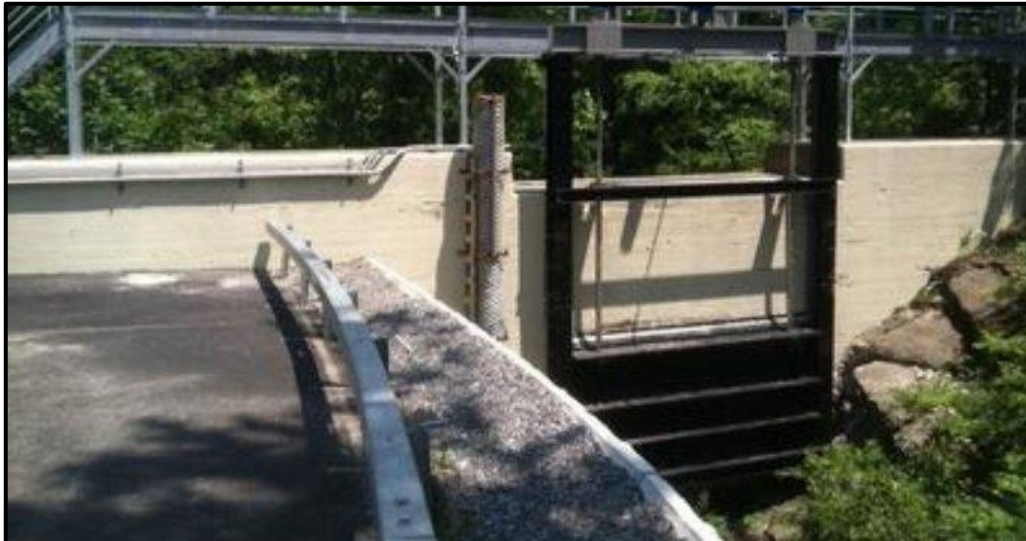
Figure 9: Downstream view of the Bowman Avenue Dam.
