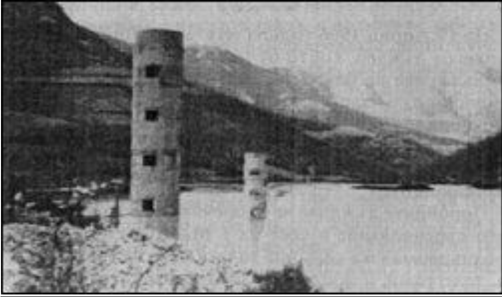
Figure 20: Photograph showing outlet spillways of the sedimentation basin [45].
