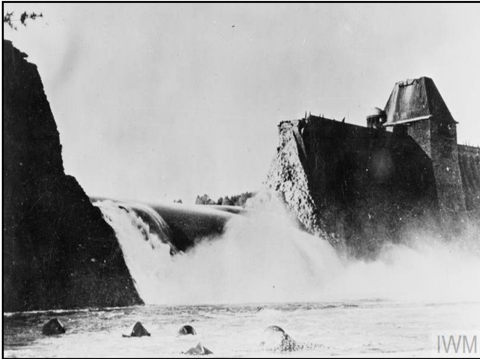
Figure 13: View of the Möhne dam breaching [23].
