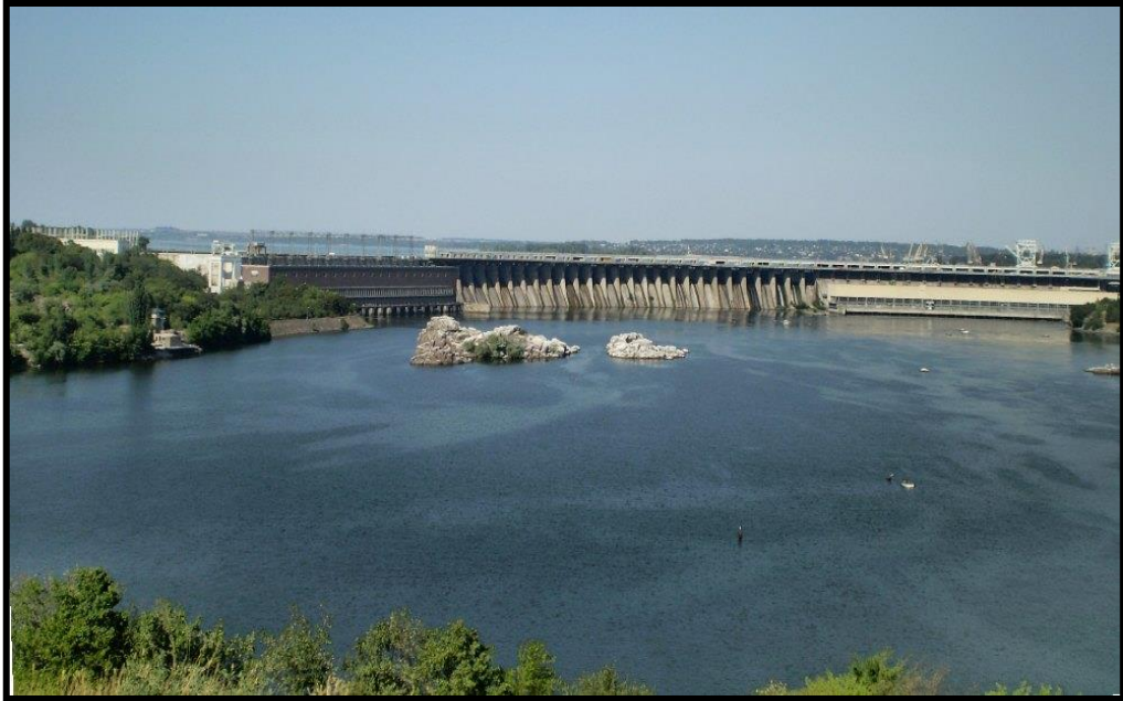
Figure 17: The dam after modernization [27].
