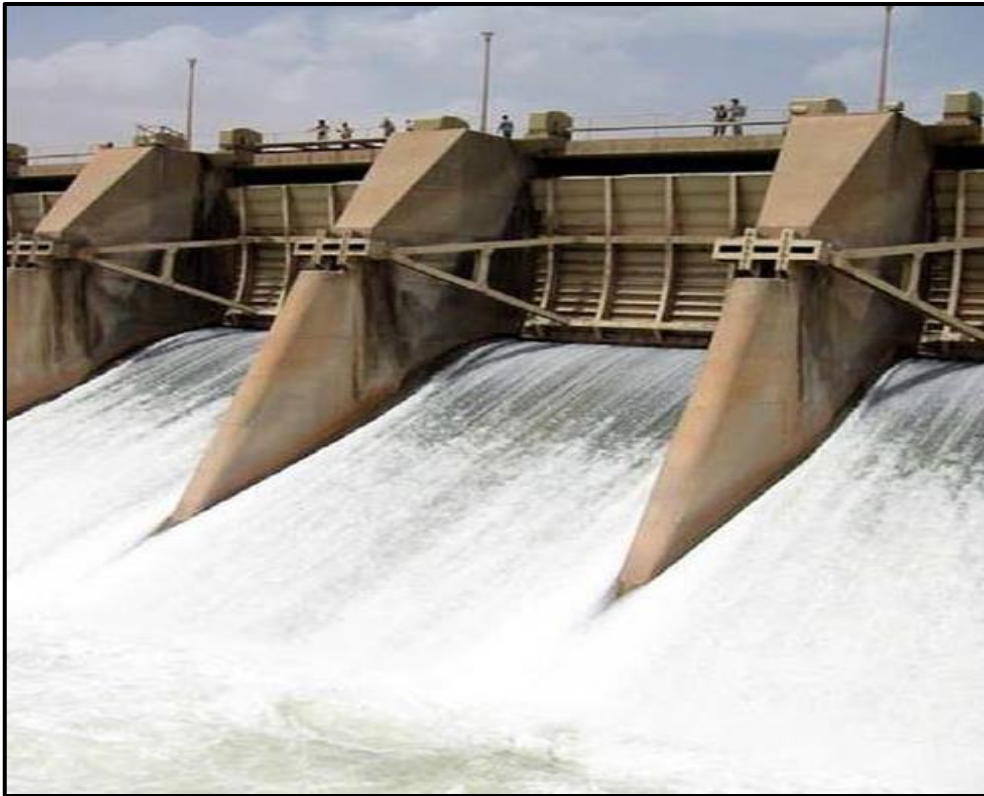
Figure 1: Dibil Dam in Iraq [7].
