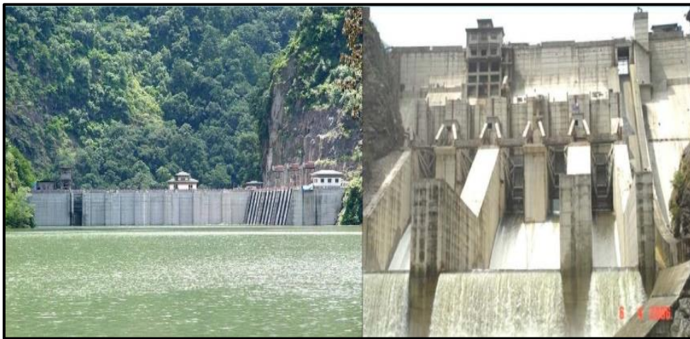
Figure 20: Upstream (Left) and downstream (Right) views of the completed dams [30].
