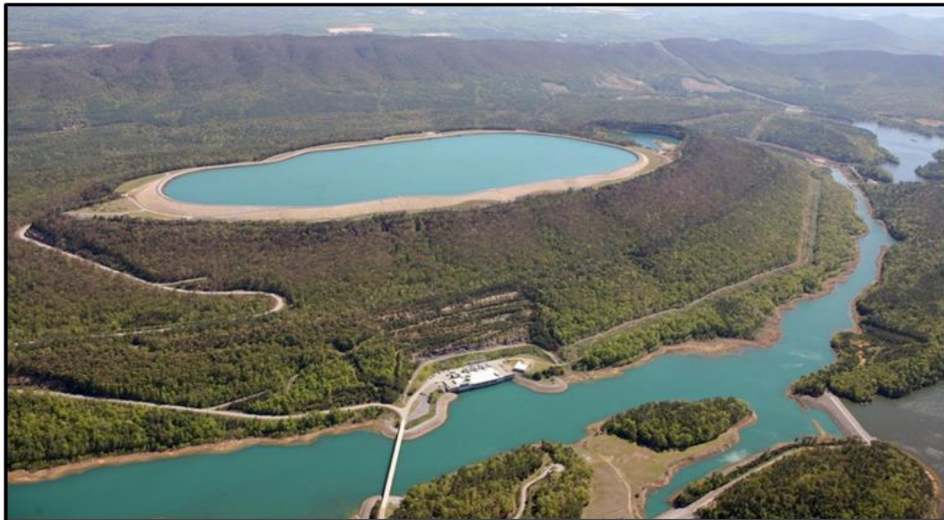
Figure 3: Rocky Mountain Hydroelectric Plant is a pumped-storage power plant.
