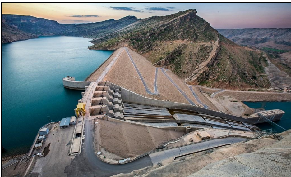
Figure 27: A view of Masjed-e-Soleiman Dam showing the rock fill dam and spillway [36].
