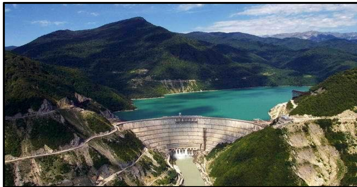
Figure 12: View of Enguri Dam, Georgia.
