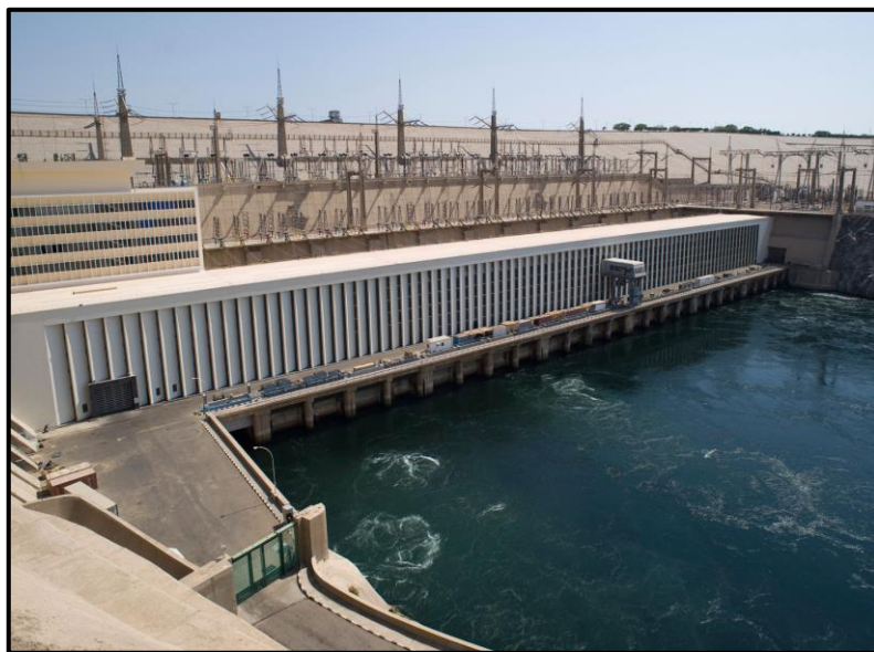
Figure 7: Downstream view of the power station at High Aswan Dam [15].
