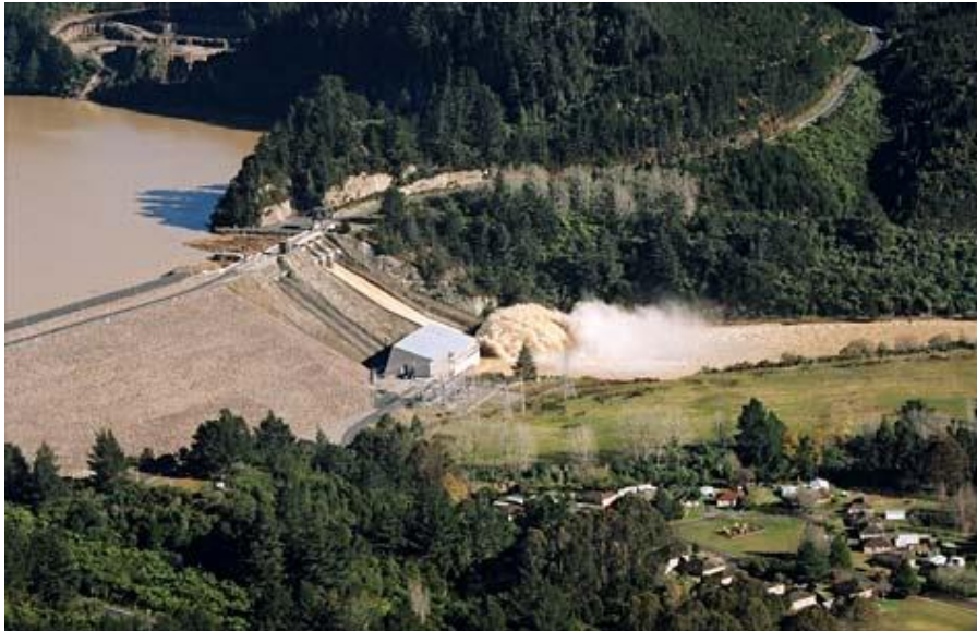
Figure 16: View of Matahina Dam [20].
