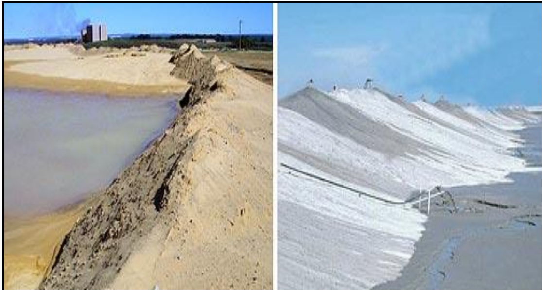
Figure 6: Loss of freeboard (left), and high freeboard (right). (© Jon Engels, Right picture courtesy of Anglo American) [25].
