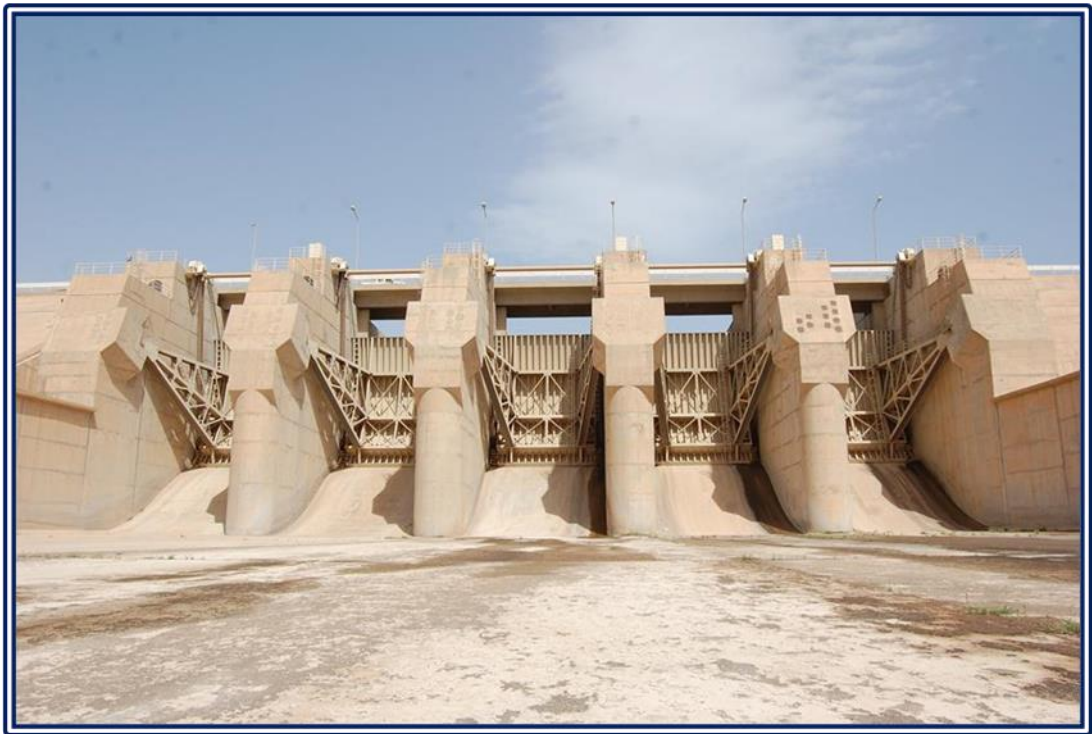
Figure 14: Spillway gates of Hemrin Dam, view from the downstream (MoWR n.d.).
