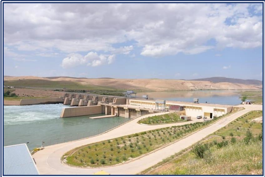
Figure 2: General view of the Regulation Dam, Mosul Dam project (MoWR n.d.).
