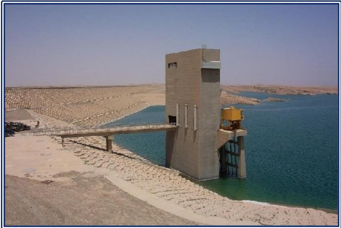
Figure 9: Adhaim Dam general view for the dam body intake structure (MoWR n.d.).
