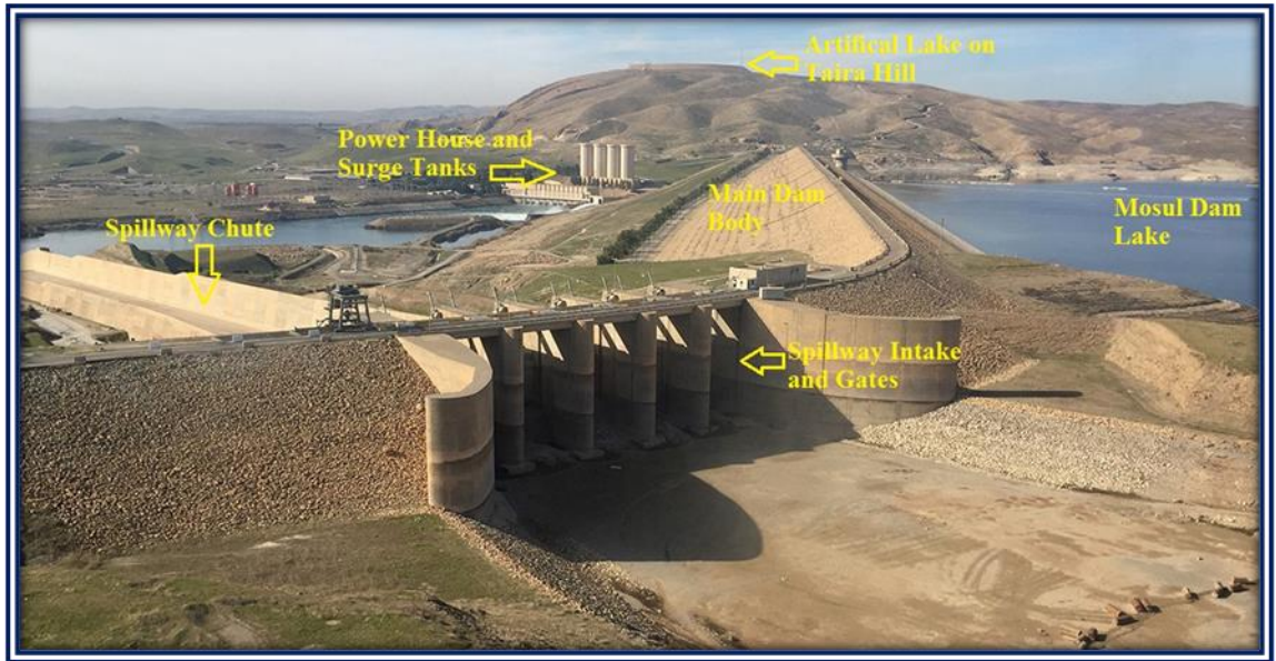
Figure 1: General view of Mosul Dam (Edited by Author). (“Trevi Group Website” n.d.).
