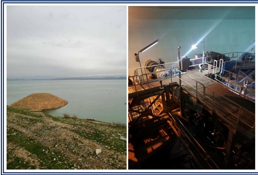
Figure 31: The main pumping station of North Jazeera Irrigation Project. a) Right: The image of the pumping station from the outside is stacked above with stone to resist the buoyance force of the water. b) Left: A picture of the pumping station from the inside (MoWR n.d.).
