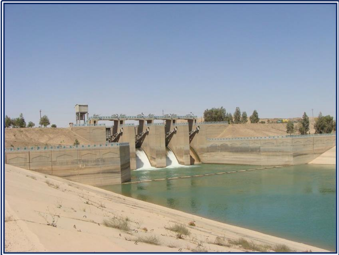
Figure 22: Downstream view of drop regulator on the Tharthar-Tigris Canal (MoWR n.d.).
