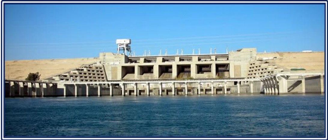
Figure 16: Concrete Section of Haditha Dam, view from the downstream (MoWR n.d.).
