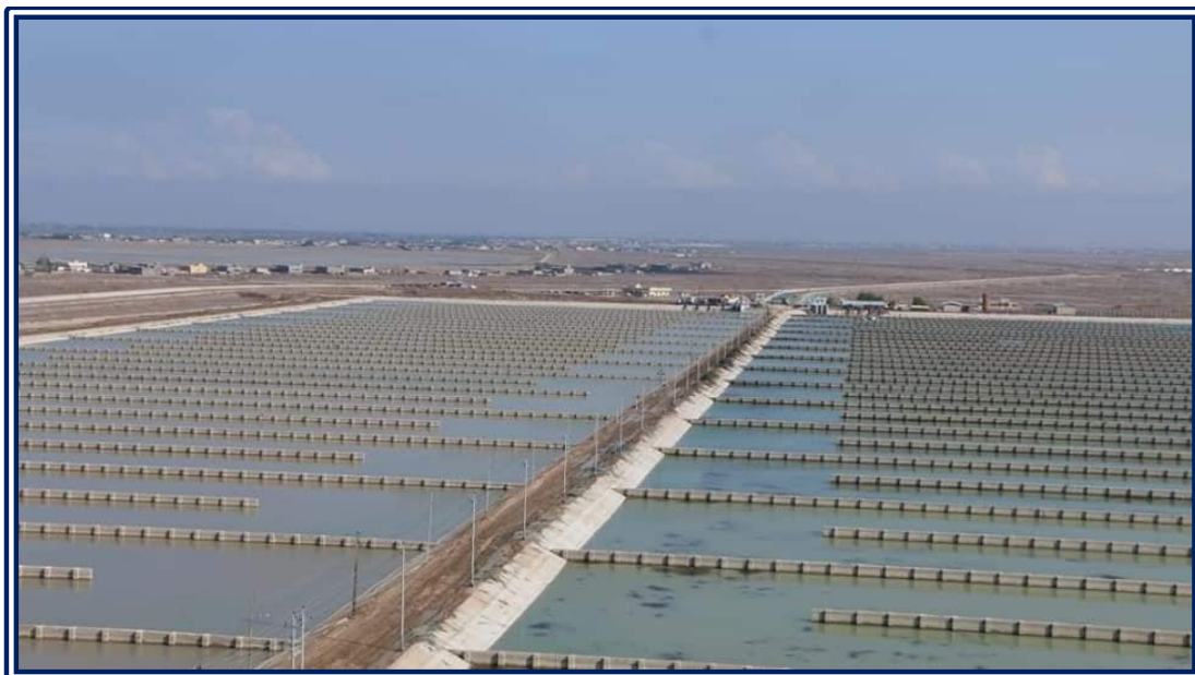
Figure 34: General view of R0 reservoir (MoWR n.d.).
