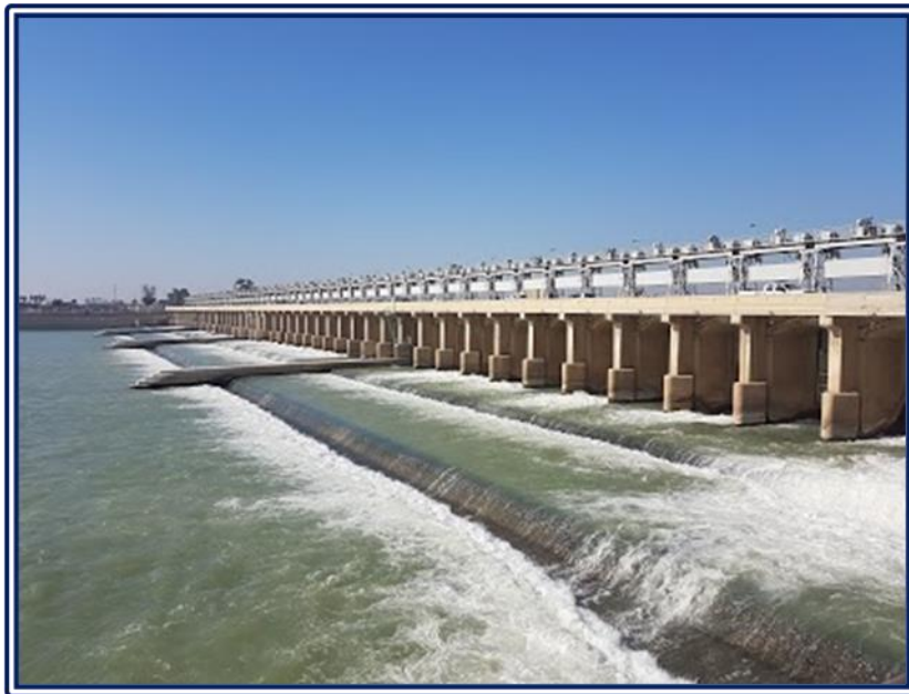
Figure 27: General view of Kut Barrage (MoWR n.d.).
