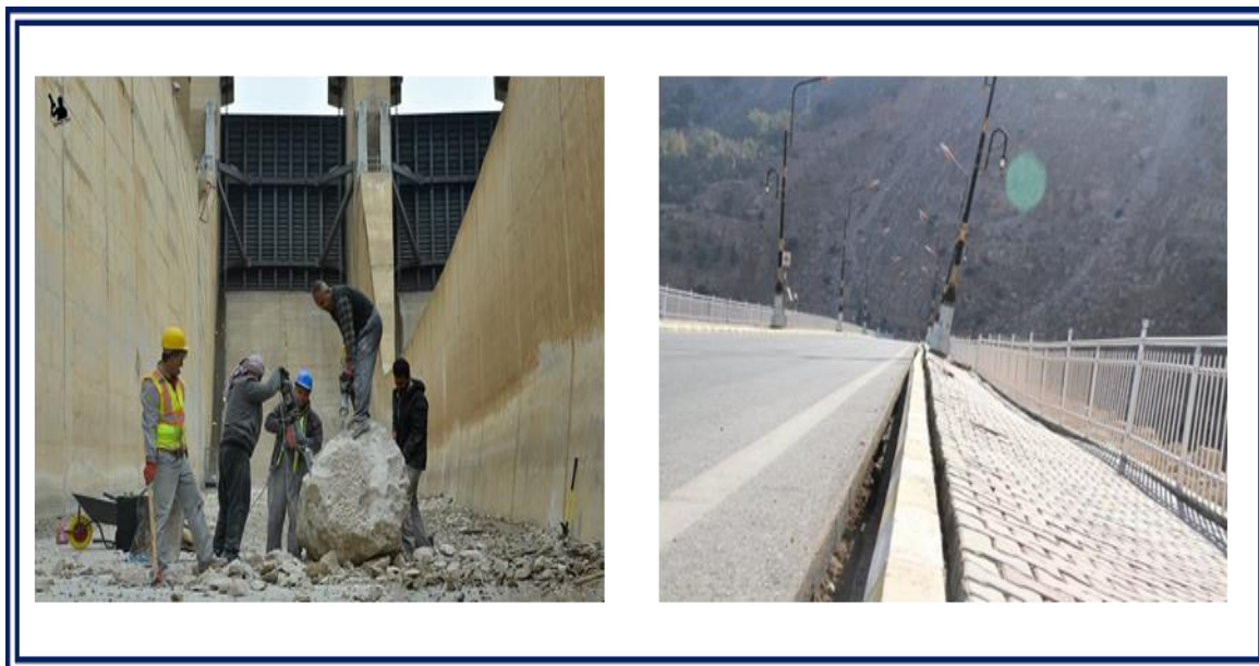
Figure 12: Aftermath of the earthquake in November 2017 at Darbandikhan Dam; a) Right: cracks in the main dam body b) left: group workers are demolishing a stone that fallen in spillway chute from the adjacent mountain. (“Darbandikhan Official Account on Facebook”n.d.).
