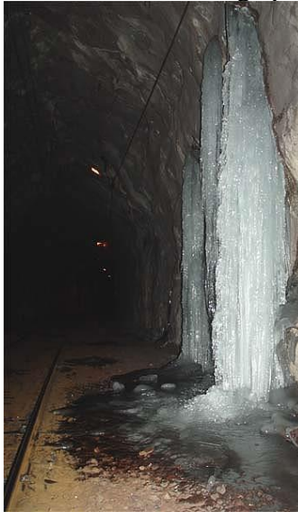
Figure 10: Ice pillar, Nuolja chainage km 1512+284 right, 2004-12-07 (Andrén, 2008).
