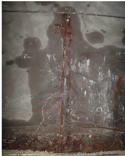
Figure 7: Drainage pipe at chainage km 1512+610, Nuolja 2004-10-07 (Andrén, 2008).
