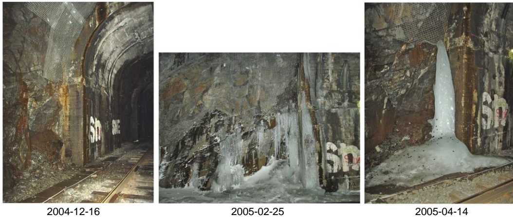
Figure 30: Difference between the three inspections, Rönninge South chainage km 29+710 left (Andrén, 2008).
