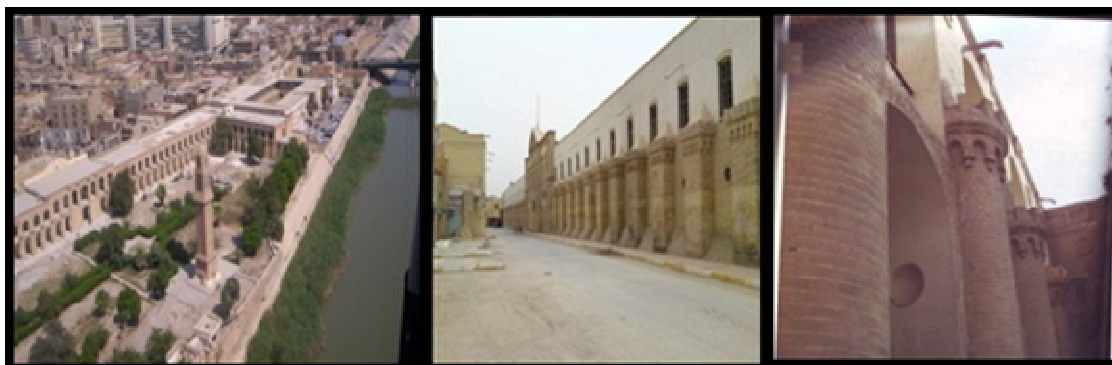
Figure 11: Qishla building like Italian design [15]
