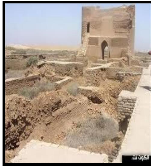
Figure 10: Photo for Gate of Wasit City
