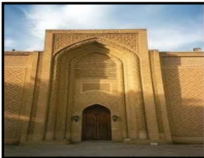
Figure 17: The Entrance of Kwled Palace, [26]
