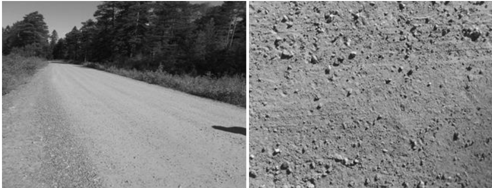
Figure 2: a: The unpaved road in Hertsö, b: The road surface
