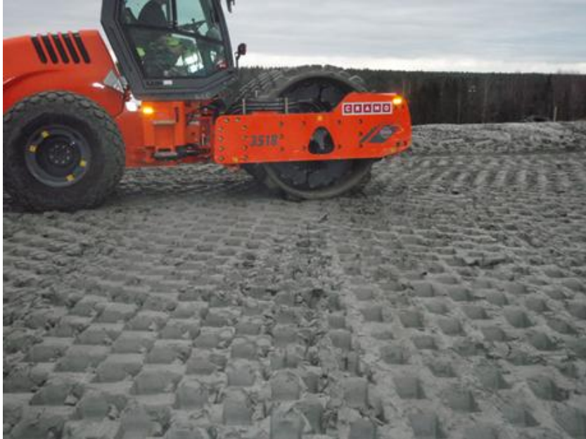
Figure 5: Padfoot compaction with 19 t roller.
